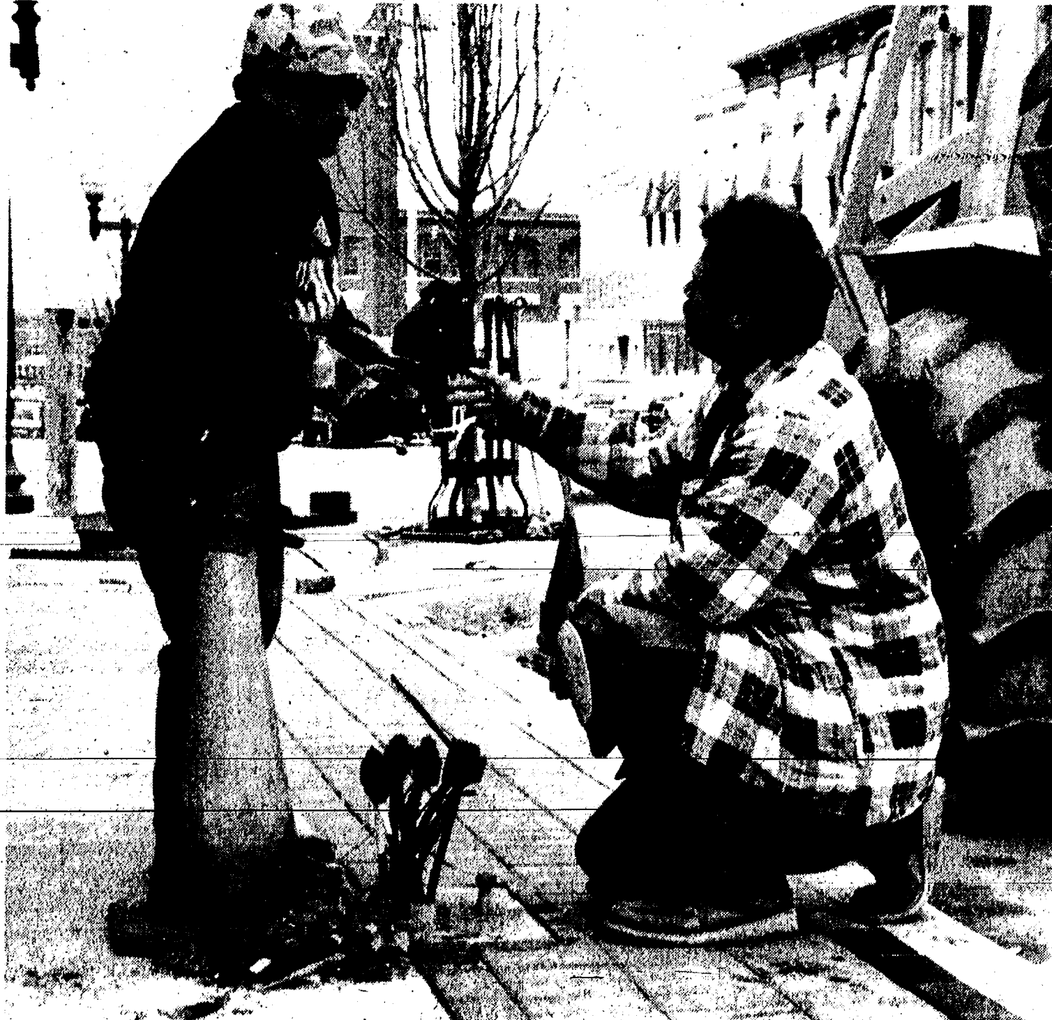
WORK HAS STARTED AGAIN on Chelsea's downtown streetscape project. Flat Rock Construction Co. plans to finish brick work on Main St. before moving on to heavier work on the side streets. The entire project is scheduled to be completed in June.
